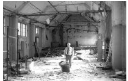
Old building with plans to covert into an Evangelical Church
